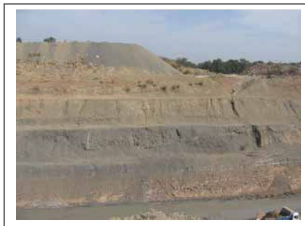
Picture 3 Excavated section showing carbonaceous shale
