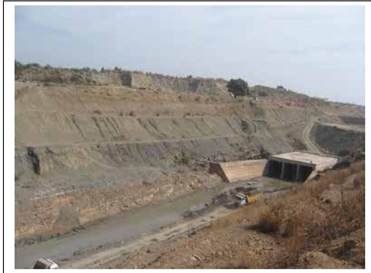
Picture 4 Cut & cover duct under construction in problematic stage
