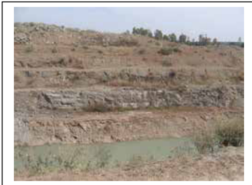
Picture 1 & 2 Excavated section showing sandstone- shale layer
