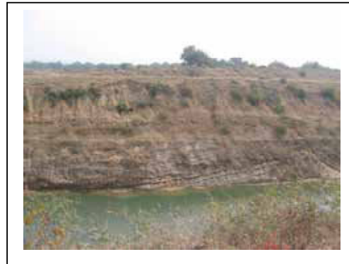
Picture 1 & 2 Excavated section showing sandstone- shale layer
